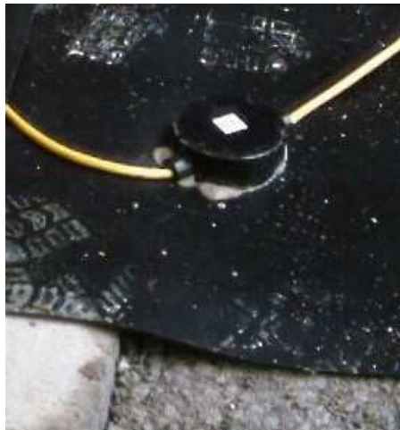
WRONG LAYING – Membrane astride a step
