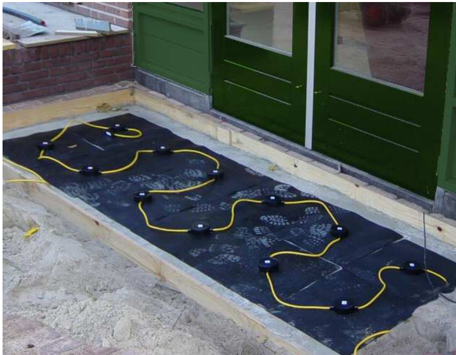
Protection of door window and glass door
